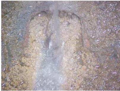
Figure 1: Sewer line filled with restaurant grease.
