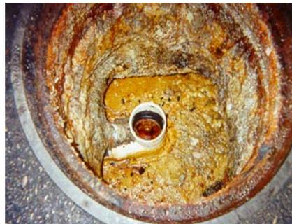
Figure 4: Clogged pipe due to FOG.
