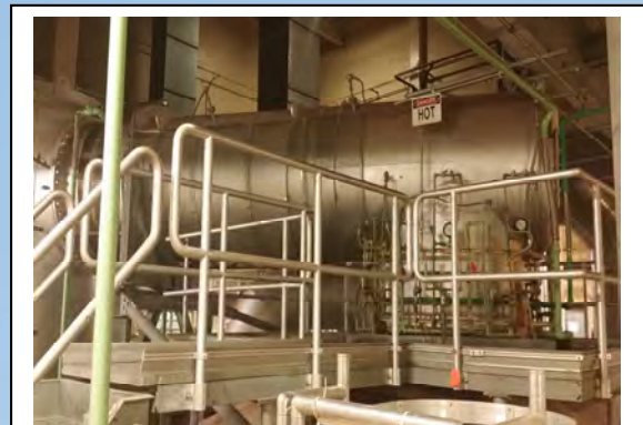
View at top of incinerator where exhaust gases first exit the reactor.
