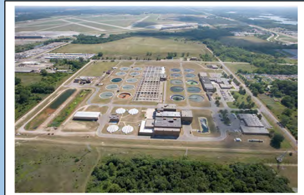
Aerial View of YCUA Wastewater Treatment Plant
