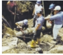
Service Crew repairing a water main
