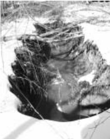
*Sewer Main collapse causing exposure of raw sewage requiring emergency repairs in 1999.*
